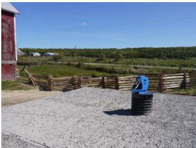
Nose pump on concrete pad
